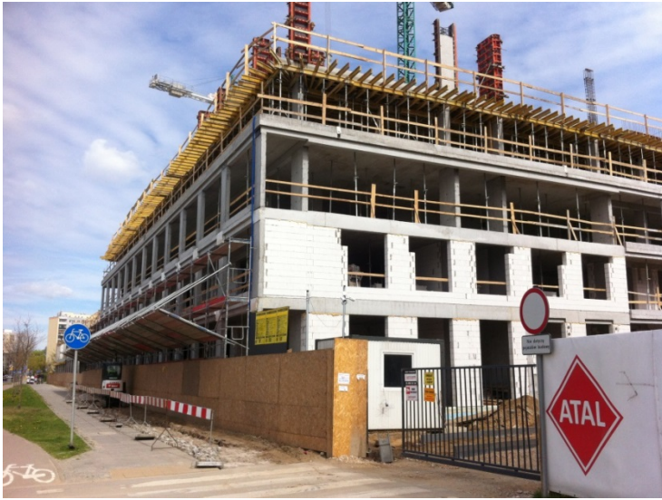
Atal's construction site in Warsaw. ©LeidenAsiaCentre
